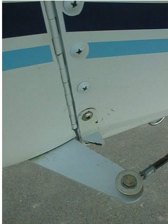
Fig 10. Photo of starboard rudder stop.
